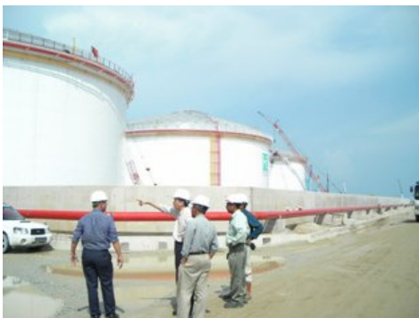
Security consultants conducting an industrial site survey
